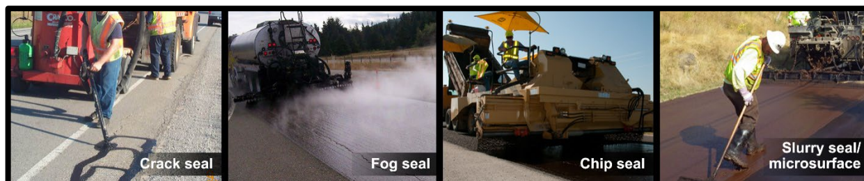
Figure 4: Examples of Capital Preventive Maintenance Treatments.
